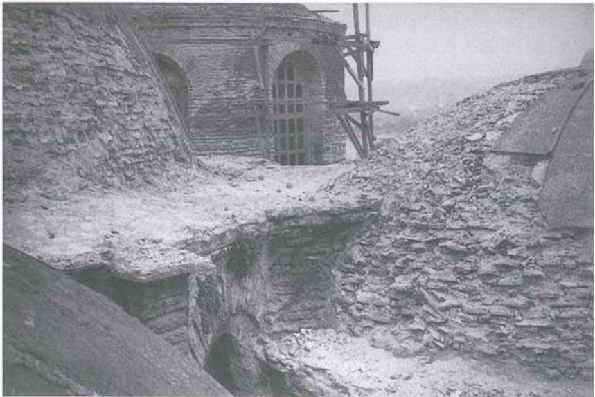
Figure 6. Zeyrek Camii, funerary chapel, the irregular brickwork of the domes (A. Neftçi, 1997).
